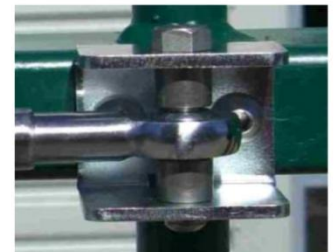
Gate bracket with spacers and gate closer attached
